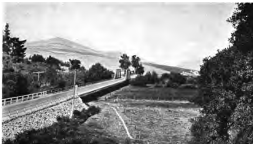
Same bridge as above completed.
